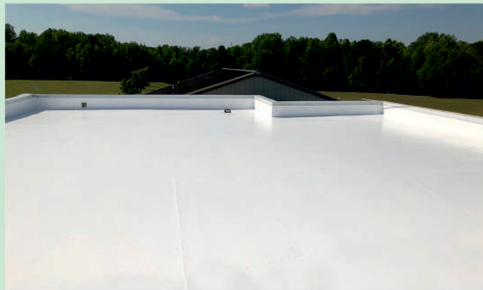
Roof of the Residential Houses
