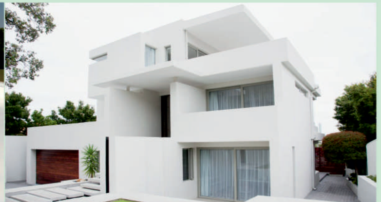
Walls of the Residential Houses
