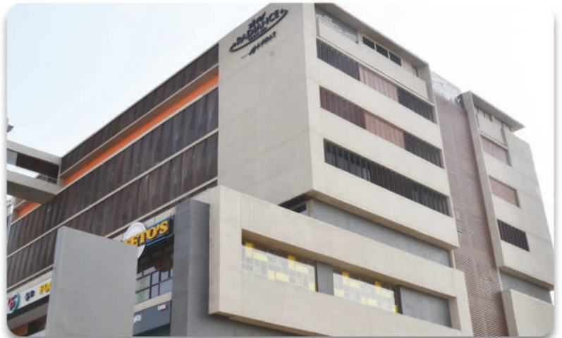
Silver Radiance (Ahmedabad) - Product : Luxture Concrete Facades
